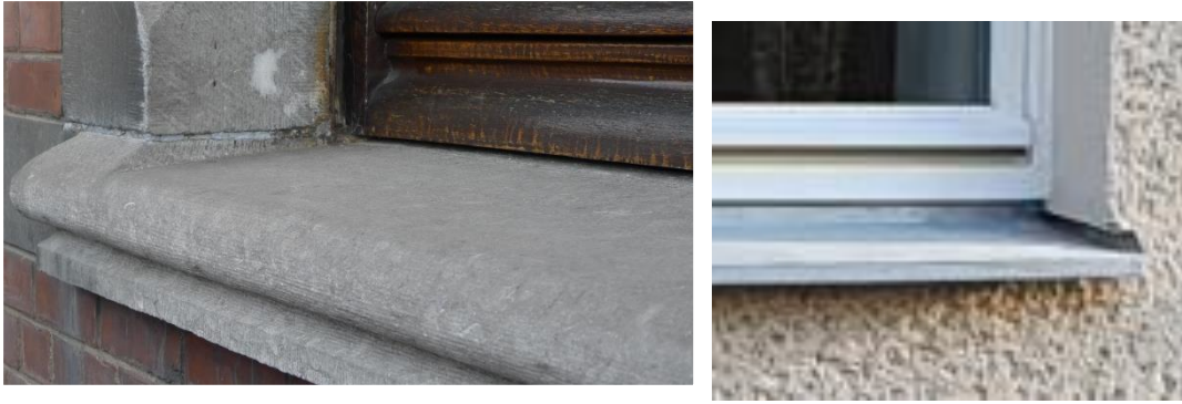
Fig. 6 Professional execution in two very different examples: Window sill in each case made of one piece (natural stone or sheet metal), window sill is inclined, protrudes from the façade, with vertical ends (not visible in the photo on the left), with drainage groove.
