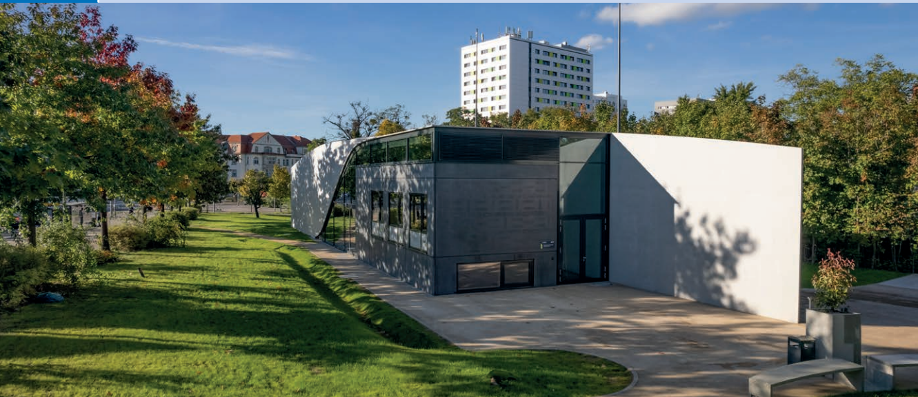
Carbonbetonhaus CUBE | Carbon reinforced concrete building CUBE | Photo: Stefan Gröschel
