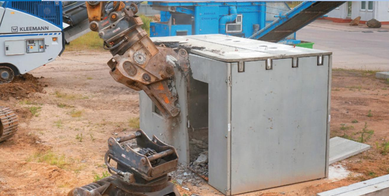
Abbruch eines Demonstrators aus Carbonbeton | Demolition of a demonstrator made of carbon concrete
