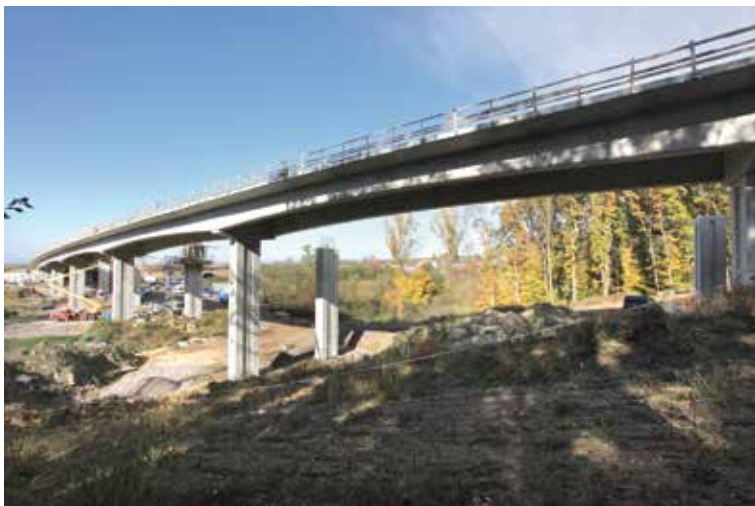
Fig. 7: Bridge across the Olichovsky Creek Valley (Photo: Jiri Dvorak)
