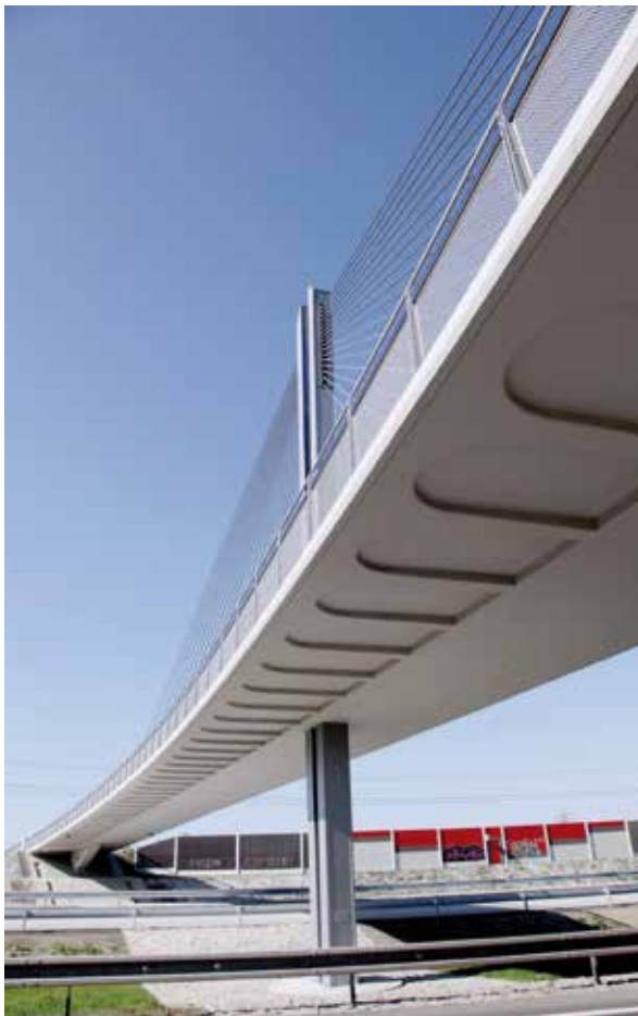
Fig. 25: Bohumin Drive Pedestrian Bridge
