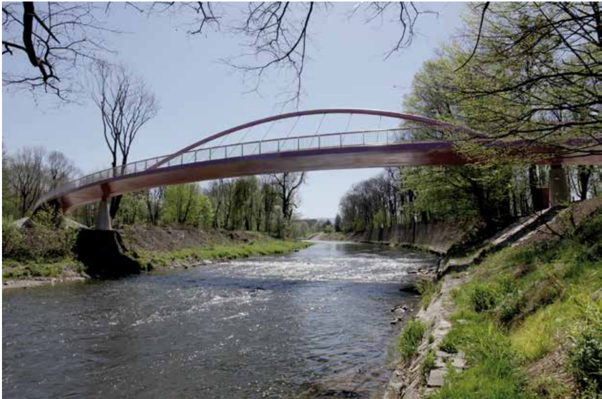
Fig. 27: Olse River Pedestrian Bridge
