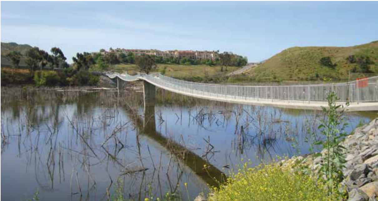
Fig. 28: Lake Hodges Pedestrian Bridge
