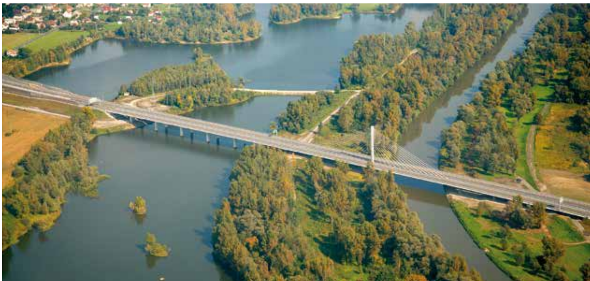
Fig. 23: Odra River Bridge
