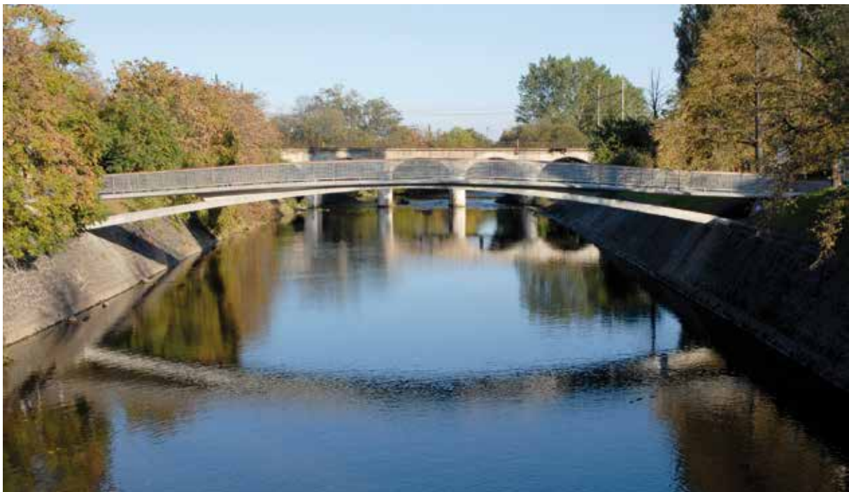
Fig. 30: Svatka River Bridge
