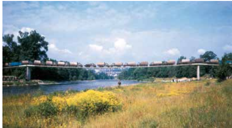
Fig. 2: Prague-Troja Pedestrian Bridge – load test (Photo: Jiri Strasky)
