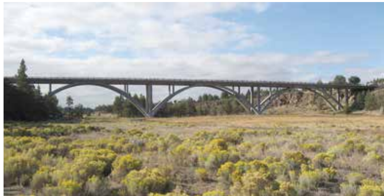
Fig. 21: Maple Avenue Bridge (Photo: Nadezda Straska)
