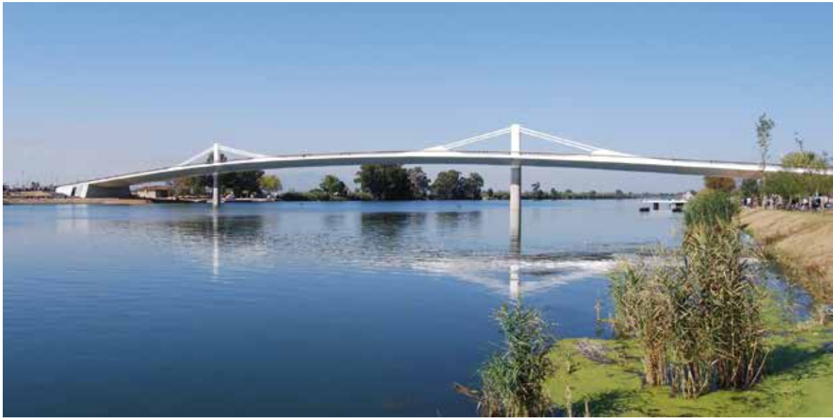
Fig. 24: Ebro River Bridge
