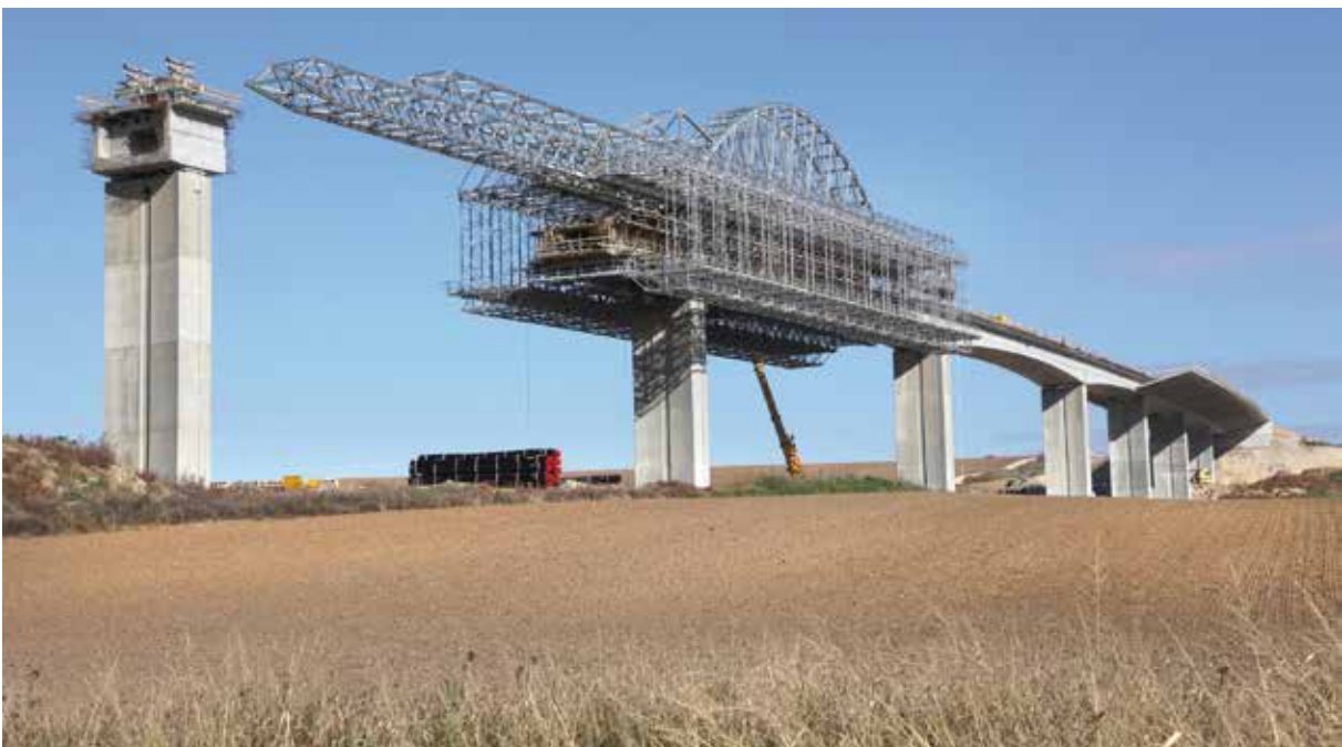
Fig. 11: Bridge across the Hostovsky Creek Valley across the Hostovsky Creek Valley
