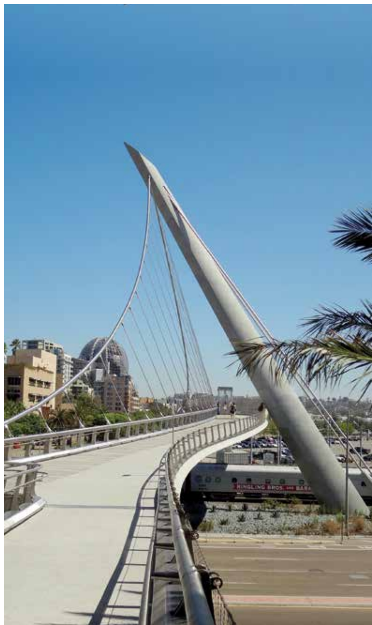
Fig. 26: Harbor Drive Pedestrian Bridge (Photo: Nadezda Straska)
