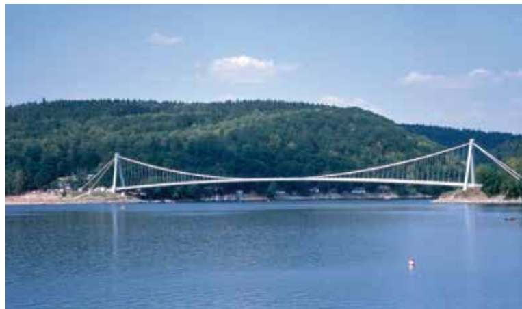
Fig. 3: Vranov Lake Pedestrian Bridge (Photo: Jiri Strasky)
