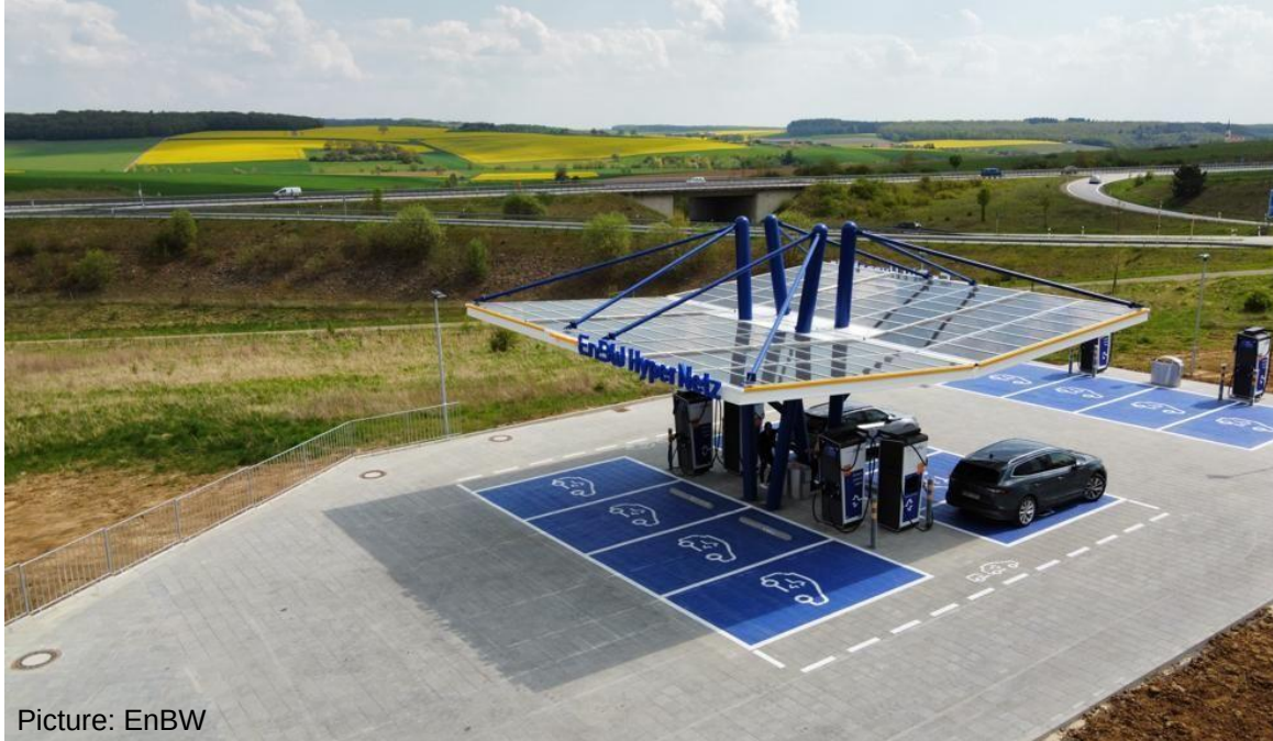
Fast charging station for passenger cars – 300 kW charging for 15 to 20 min
