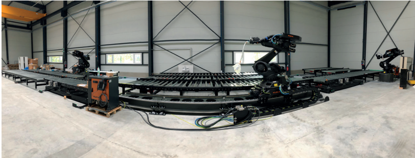
Fig. 01 CarbonConcrete Technical Center, HTWK Leipzig. *© Photo: Otto Grauer, FG Sustainable Constructing, HTWK Leipzig
